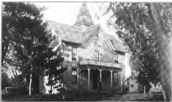
RESIDENCE OF W. A. KESTER, CENTERDALE
